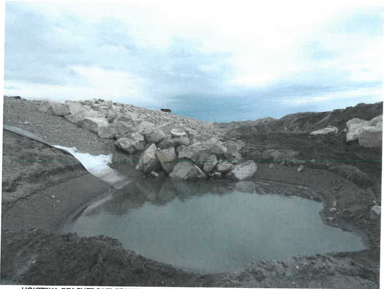
HOKITIKA BEACHFRONT SEAWALL – 27 SEPTEMBER 2013 Bottom View Looking Southwards
